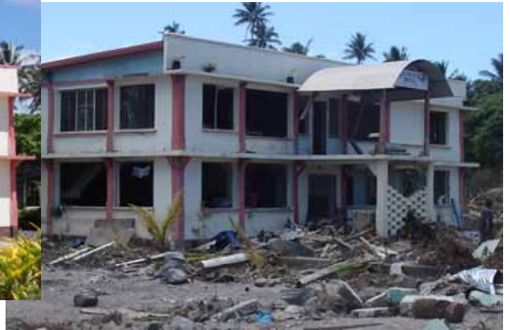
Matamatagi Motel 2 October 2009
